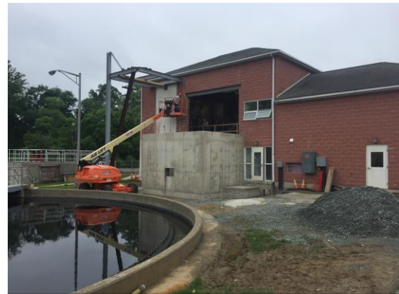
Grit System Addition
