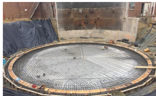
Primary Digester - Base Slab Reinforcing Steel
