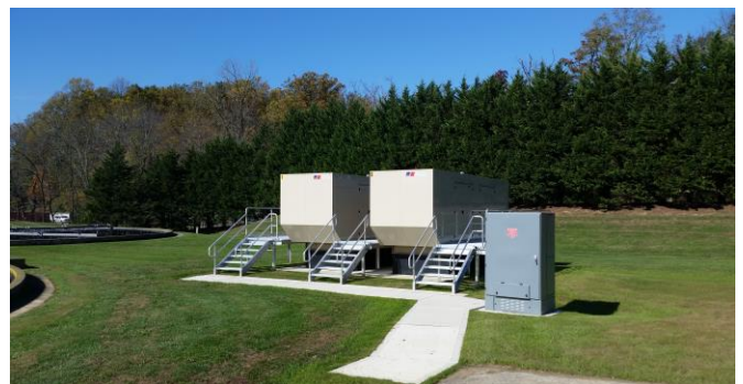
Two (2) 500kw Emergency Diesel Generators and Trvstar Permanent Docking Station at WWTP
