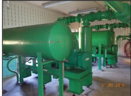
Blowers 125 HP 18 psig PD Blower 3,340 scfm
