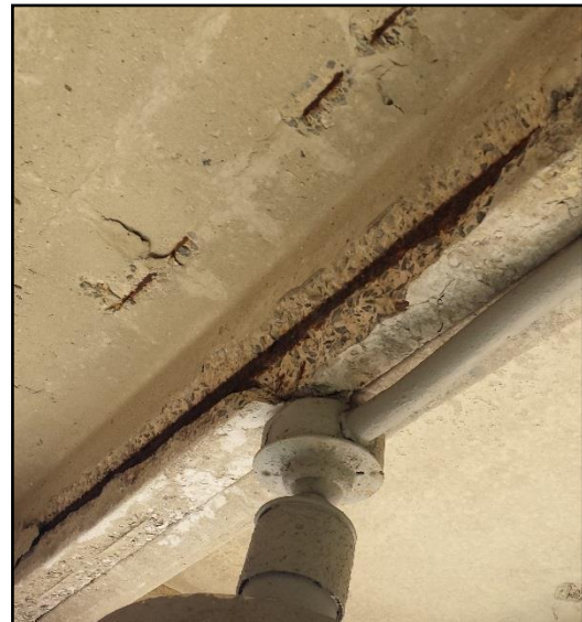
Montgomery Avenue Concrete Deterioration
