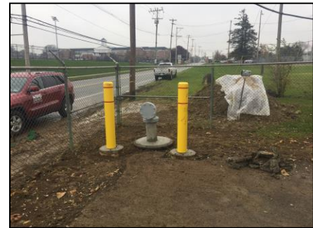
Montgomery Ave. Bypass Pump Discharge Connection
