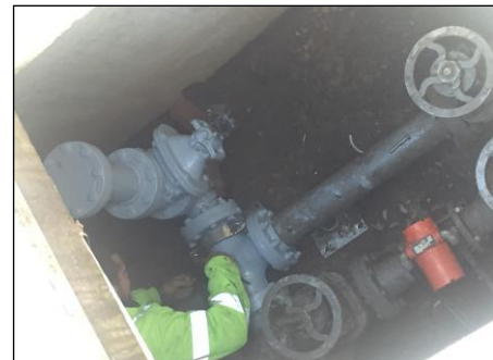
Trinity Drive Pump Station Bypass Pump Connection
