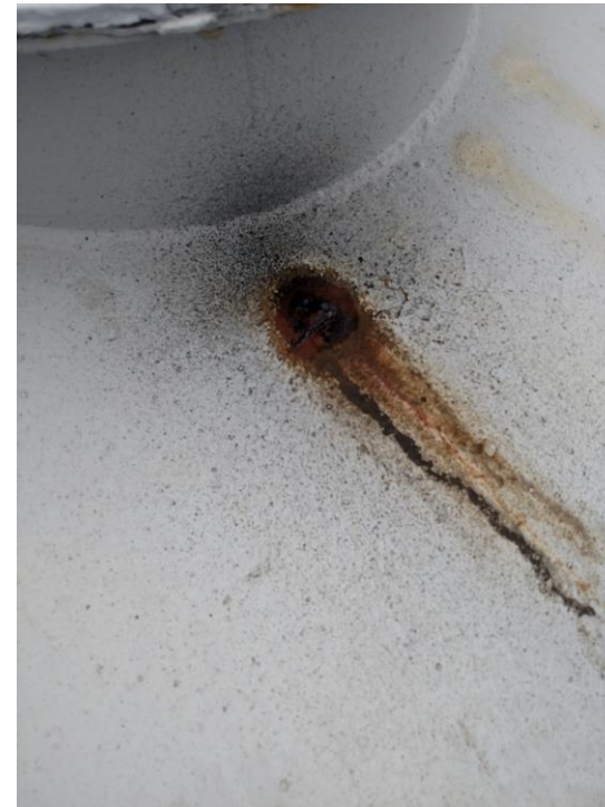
Digester Roof Gas Leak
