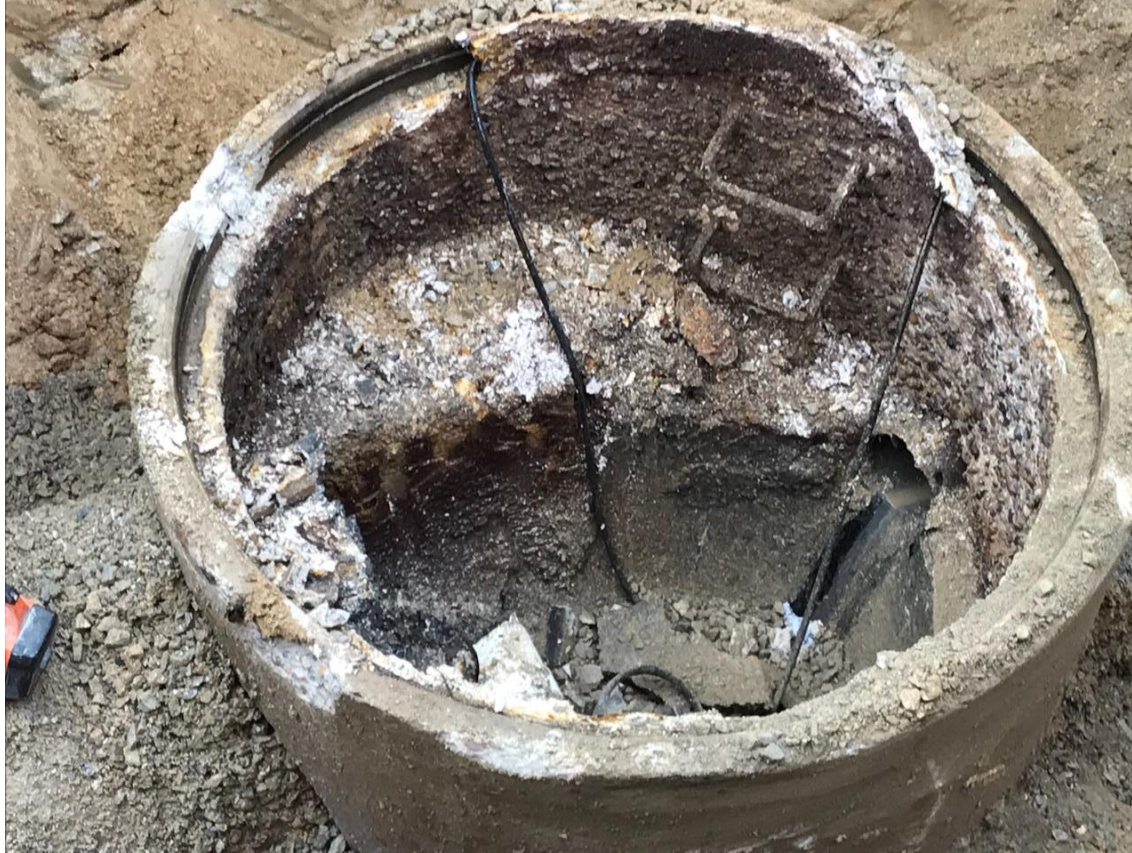
Before: Broken and Deteriorating Manhole
