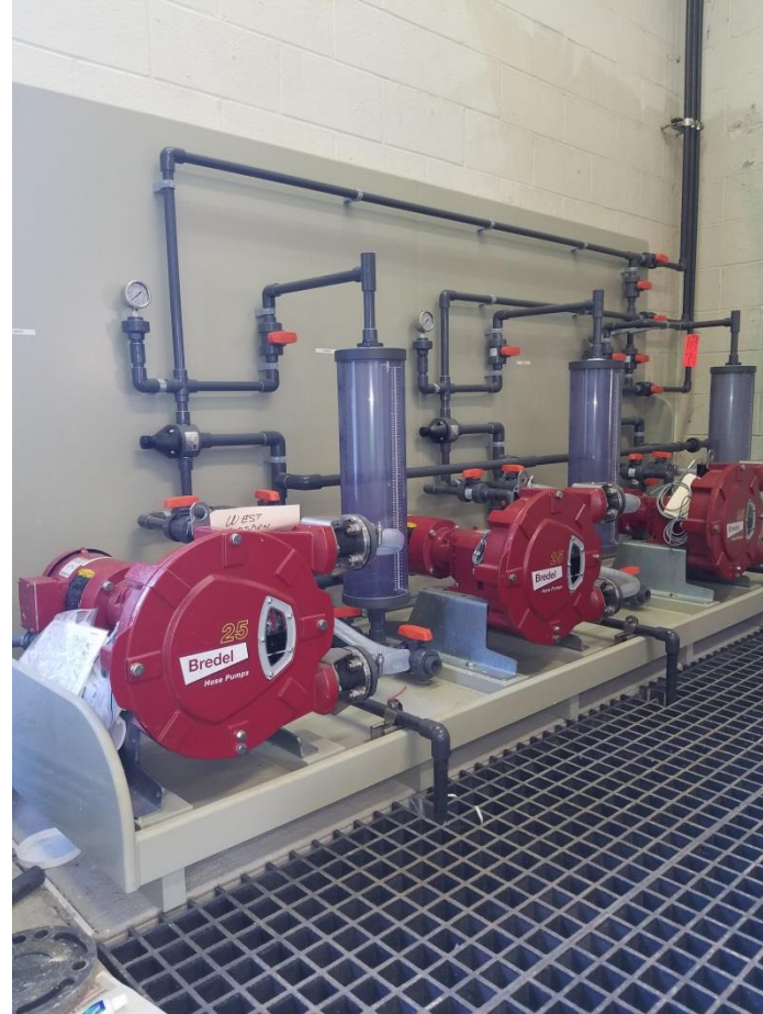
New Hydrated Lime Feed Pumps & Slurry System
