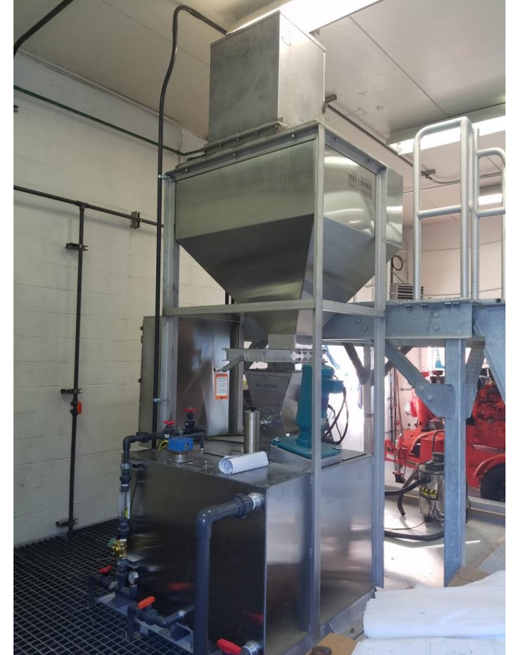
New Hydrated Lime Feed Pumps & Slurry System
