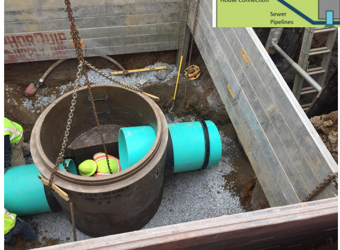
2018: New Manhole to Replace Broken and Deteriorating Manhole
