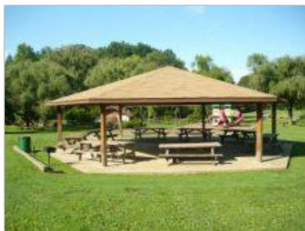
Pavilion at Barker Park (Source: West Goshen Township)
