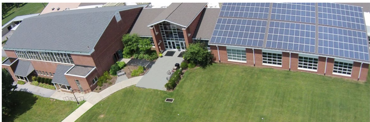
Solar PV on Westtown School Athletic Center
